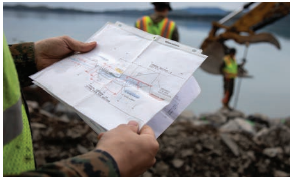
U.S. Marine Corps GySgt Tyler Brookbank, a combat engineer for the 6th Engineer Support Battalion, 4th Marine Logistics Group, Marine Forces Reserve, consults construction plans while supervising earthwork operations at Shepard Point near Cordova, Alaska, Aug. 21, 2024. Alaska National Guard photo by Alejandro Peña.
