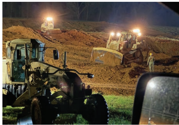
Soldiers gained mission-critical proficiency training in heavy equipment operations and logistics.
