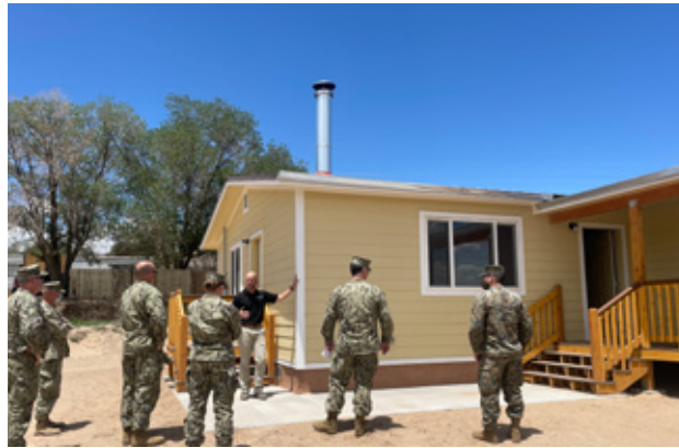
Service Members perform a walkthrough of a Navajo family house constructed during IRT's Operation Footprint mission in Gallup, New Mexico
