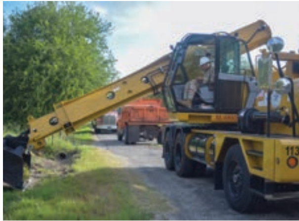
Heavy equipment operation, logistics, and mission planning were just a few of the training opportunities the FY22 civil-military partnership with Nueces County provided.
